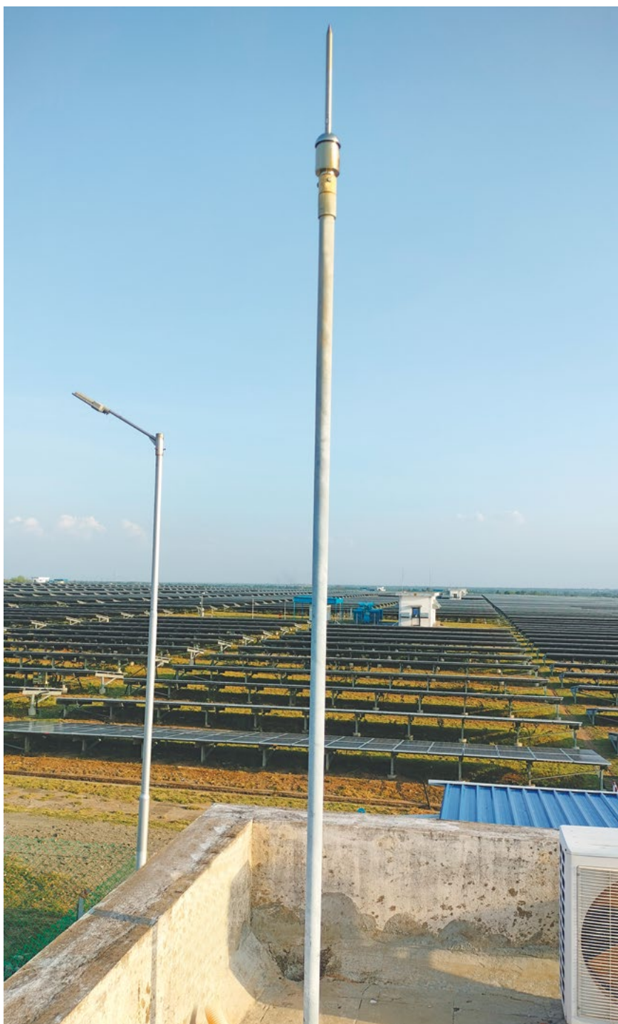
Lightning Arrester at WREL's project in Trichy district, Tamil Nadu
