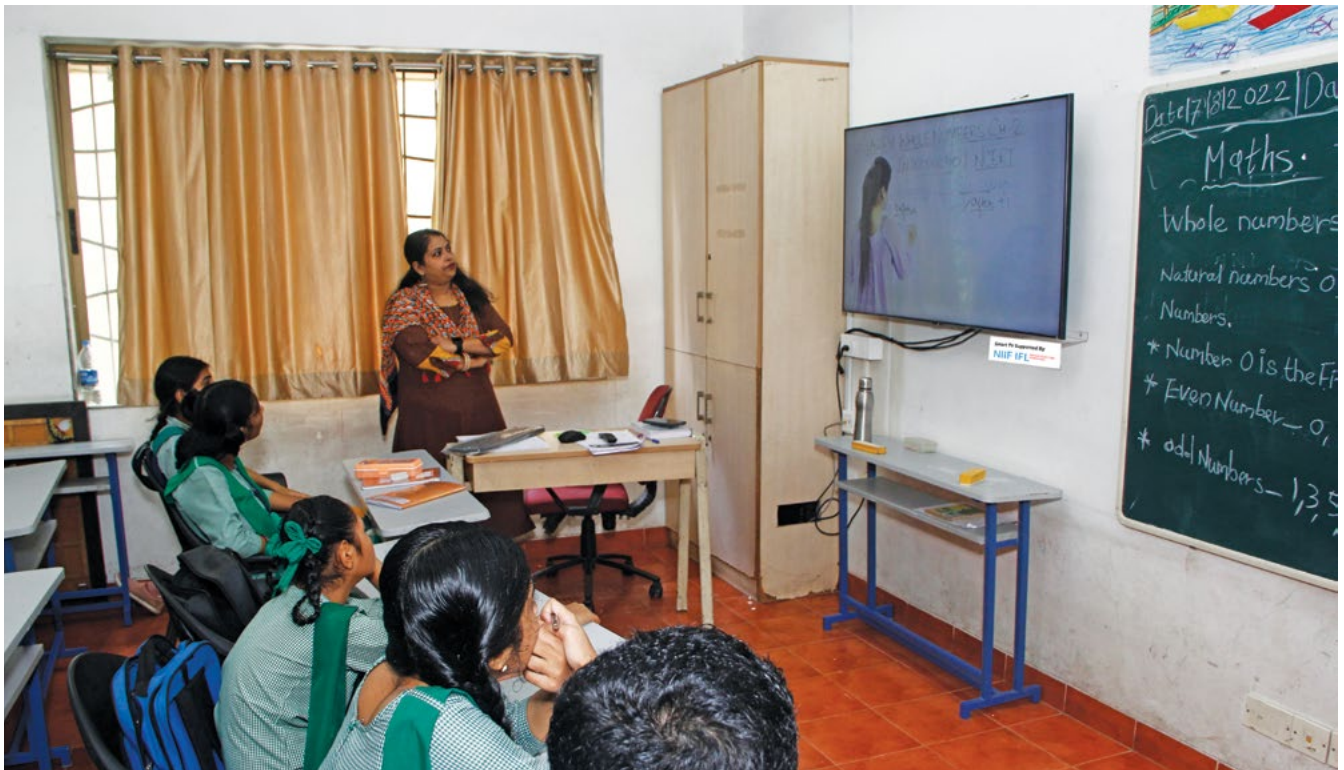
NIIF IFL has supported Vipla Foundation to provide solar power for a school (with students with special needs)
