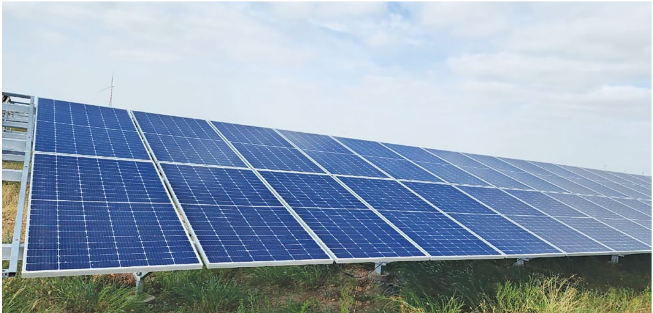
Use of bifacial solar modules at Clean Solar Power (Bhainsada) Private Limited
